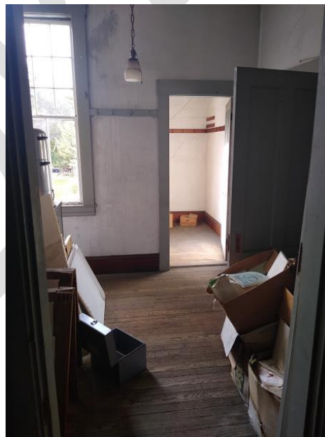
Anteroom between the Ceremonial room and the second floor hallway (may have been the original kitchen) looking west with coat room in the background
