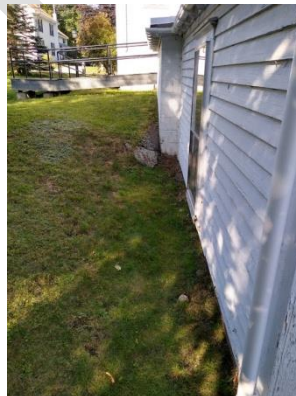
Negative grade on west side of 20 th century addition
