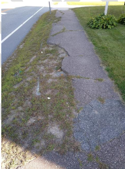
Deteriorated asphalt sidewalk
