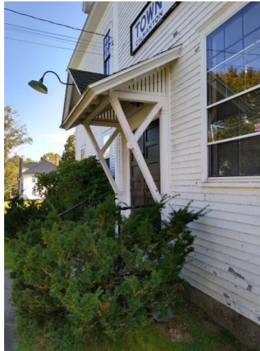
Main entry roof system
