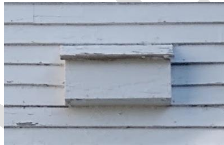
Close up on wooden cover on end of truss
