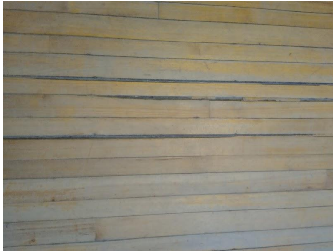
Section of auditorium flooring showing wear.
