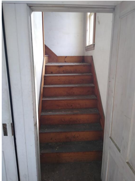
Behind the right hand hallway door is the first flight of stairs from the second floor to the third floor
