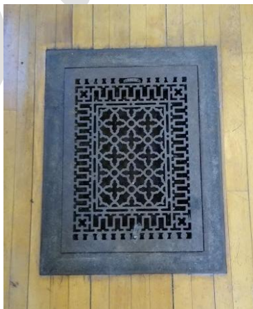
Close up of original hot air grate
