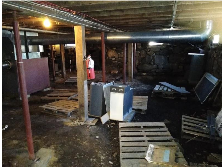
Mechanical space in basement
