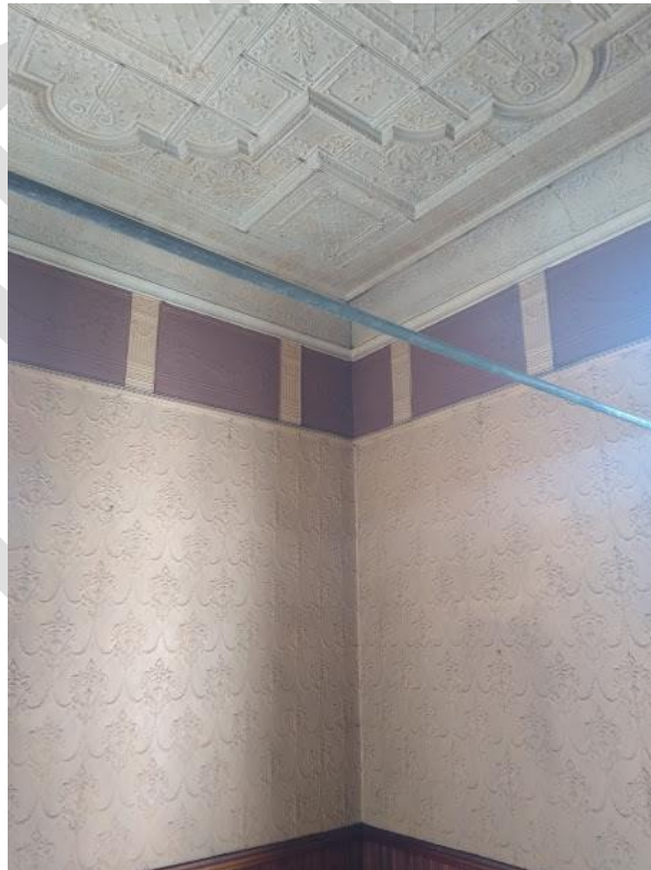
Detail of pressed tin ceiling and walls in Ceremonial room facing the northwest corner
