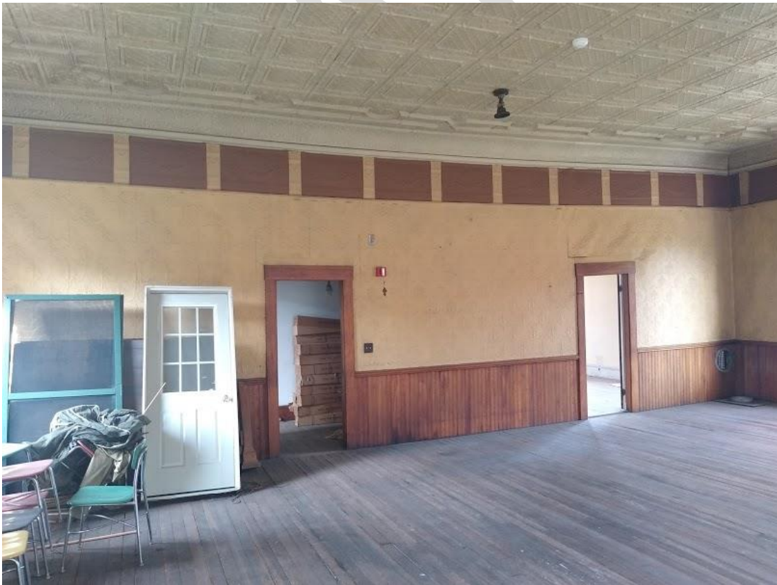
Ceremonial room looking north at sagging partition
