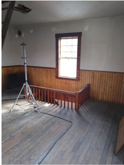
Finished tower space looking south
