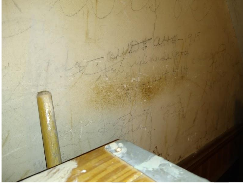
Graffiti from 1914/1915 on southerly plaster wall in ticket booth
