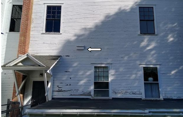
Wooden cover on end of truss on west side
