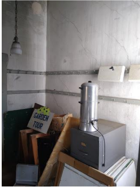
Anteroom (possible kitchen) looking south west, with stove connection on far right into exterior chimney (not seen in photo) Plaster shows stress cracks
