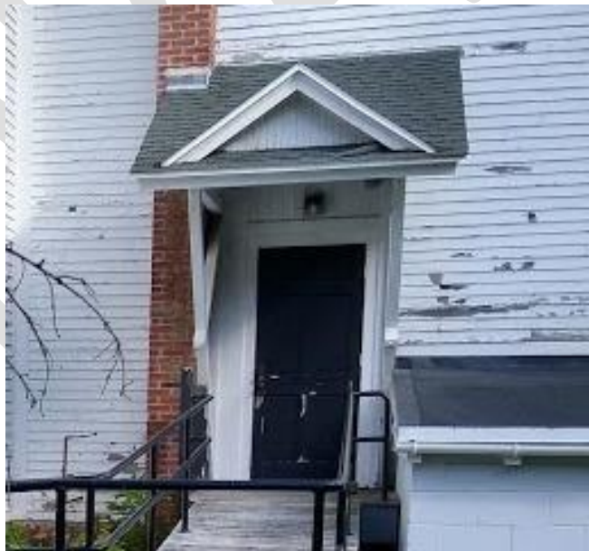
West side ADA entry roof system
