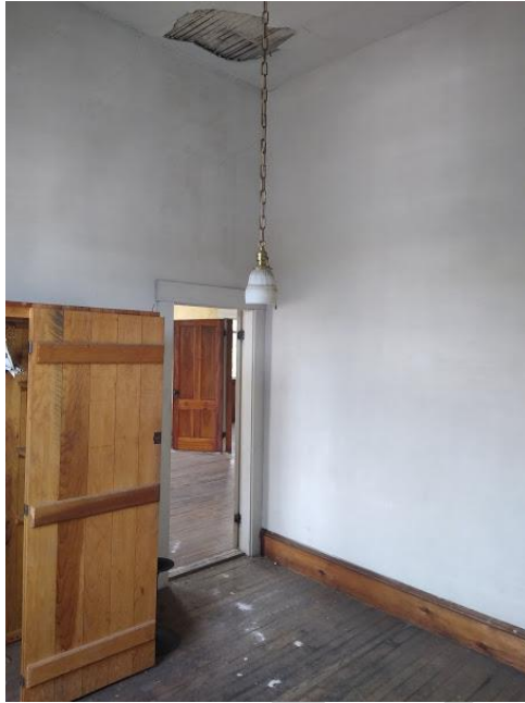
North Anteroom (Anteroom "B") looking from doorway of second floor landing Note plaster failure in ceiling
