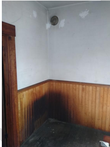
Location of kerosene stove at top of stairs
