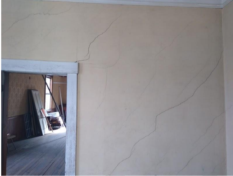
Close up of stress cracks in partition wall common with ceremonial wall Cracks and sagging of wall due to lack of support across span.
