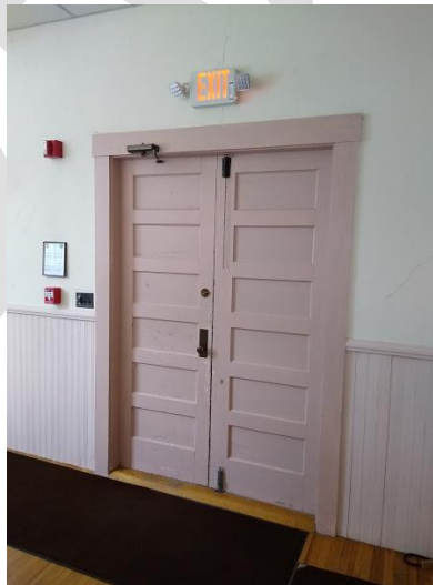
“Crash bars” will be installed on the vestibule doors
