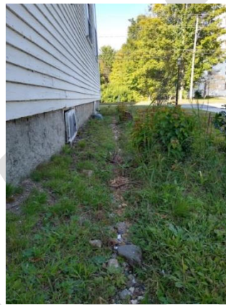
Drip line with negative grade on east side of main building
