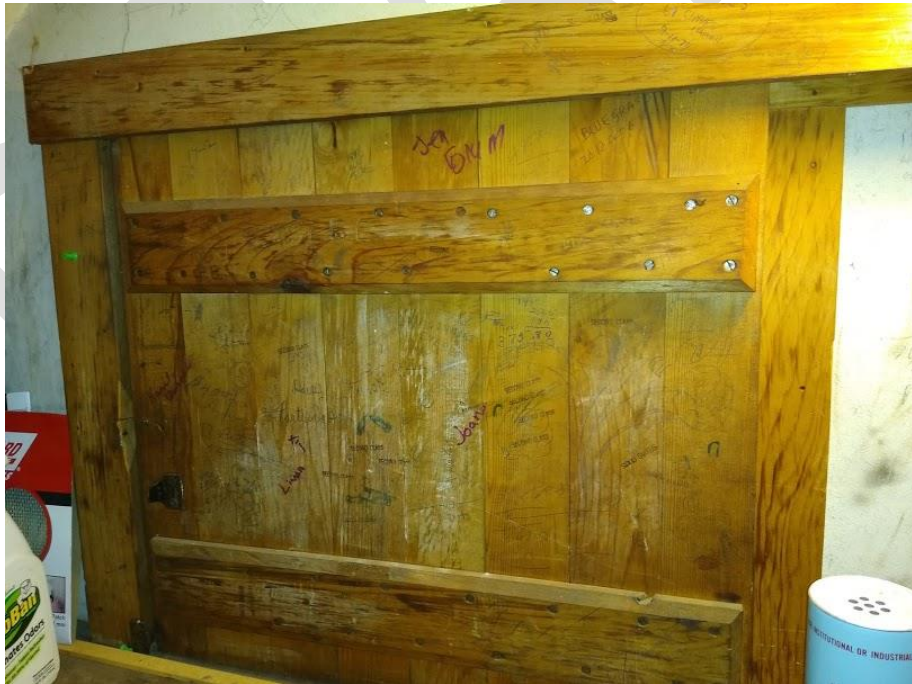
Ticket booth sliding wooden security door that covers ticket booth grate Graffiti on back of door
