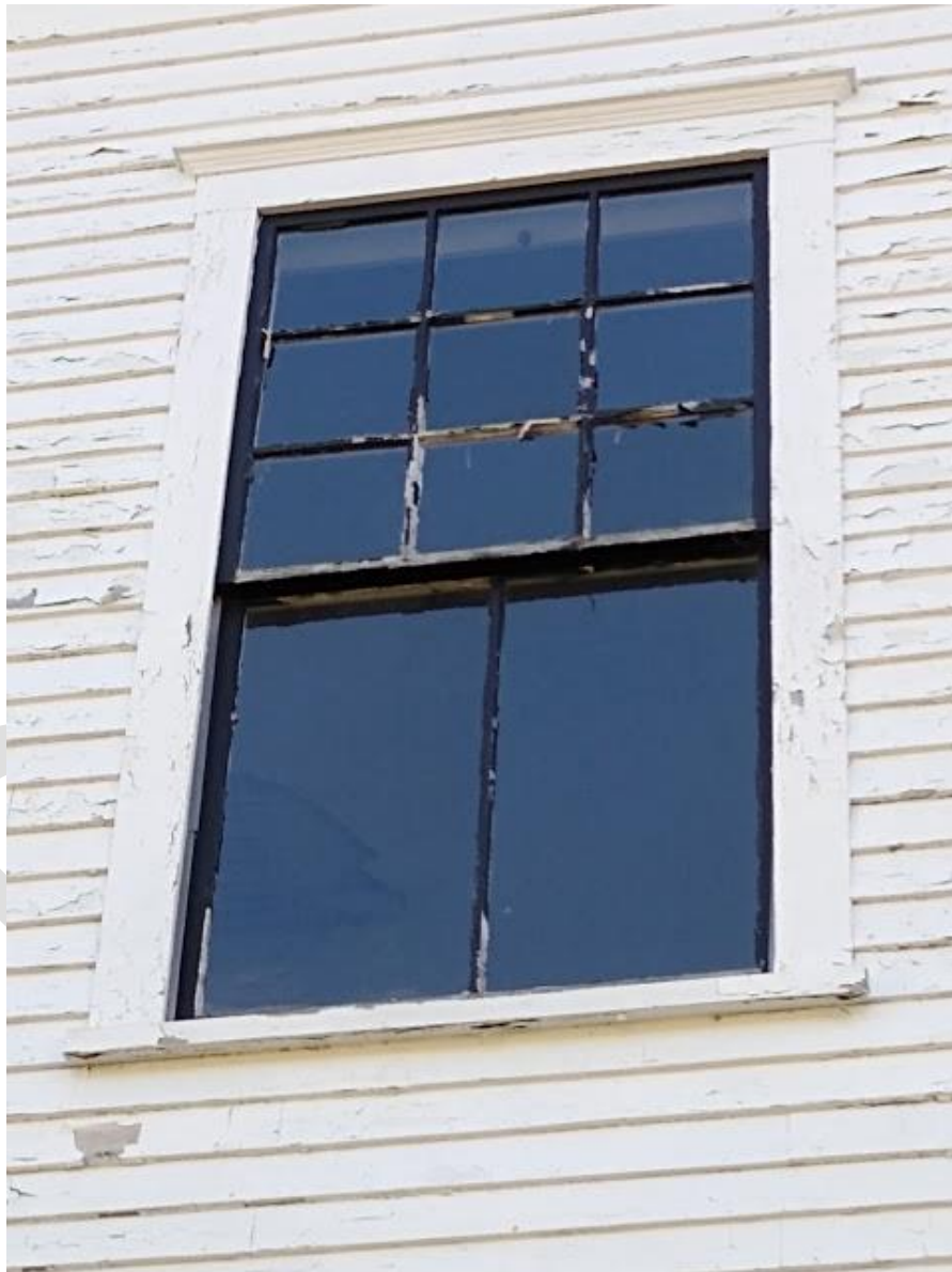
East 2 nd floor window indicative of all window conditions especially 2 nd floor, dormer and tower windows
