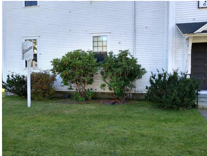
North side overgrown trees and shrubs
