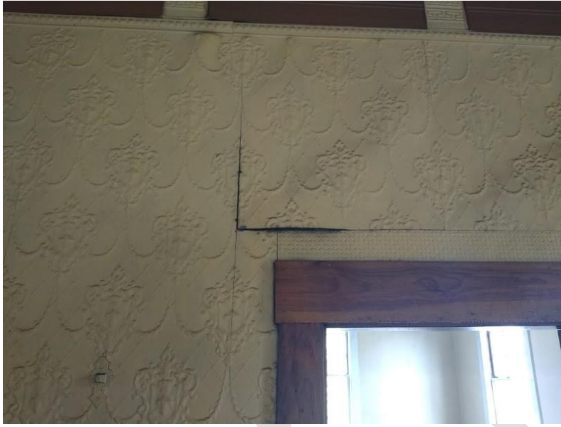
Close up of the Ceremonial room side of sagging partition wall and movement of pressed metal wall siding
