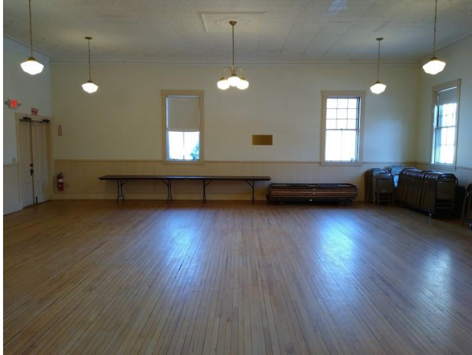
Auditorium looking north
