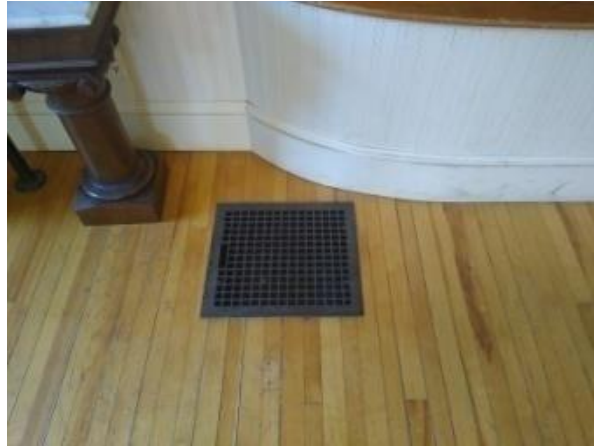
Easterly cold air return near stage
