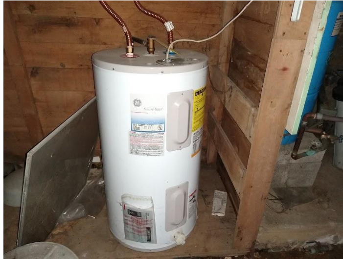
Newer water heater
