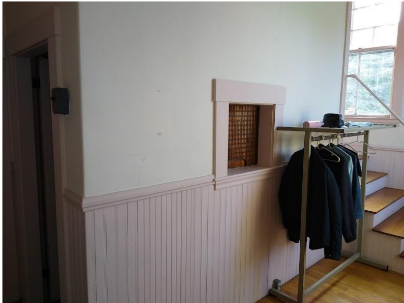
Vestibule looking south looking towards ticket booth
