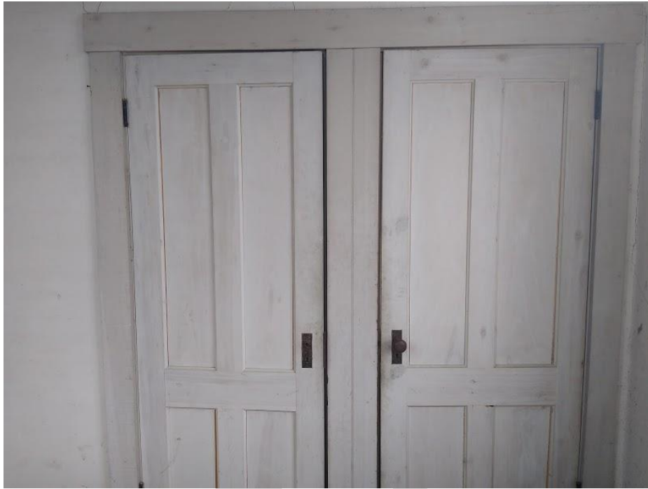
Double doors at end of hallway looking south
