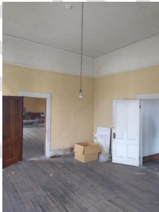
East Anteroom (Anteroom "A") looking south
