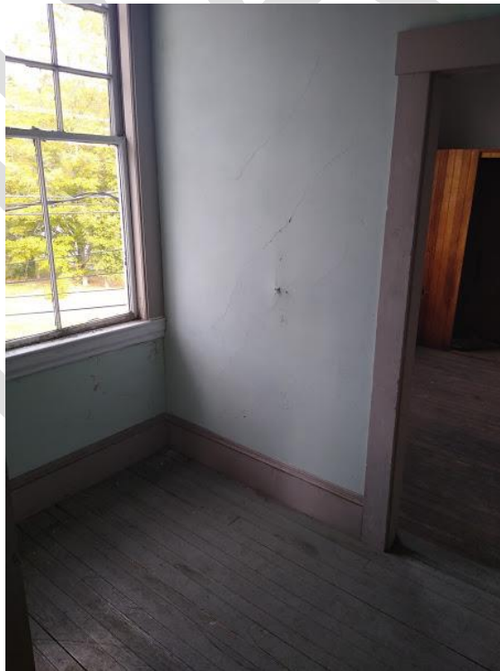
Stress cracks in plaster near doorway leading into Anteroom "B" looking east
