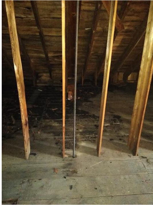
Attic looking west at metal support rod
