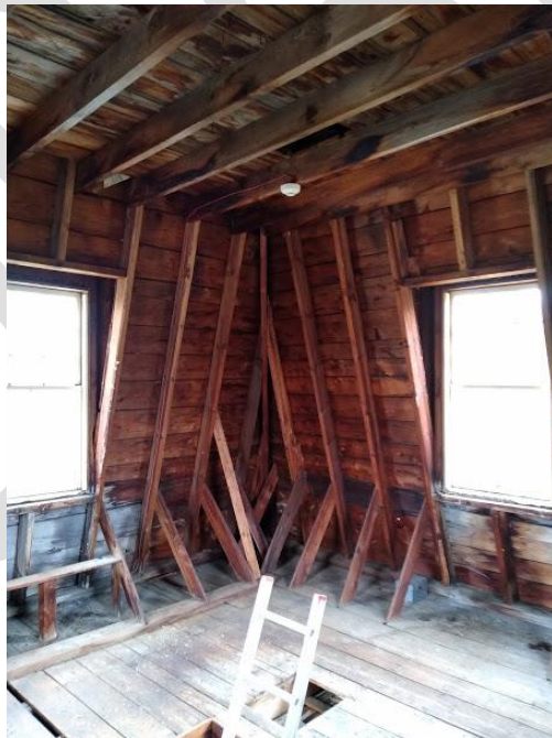
Unfinished attic space above tower room looking southeast
