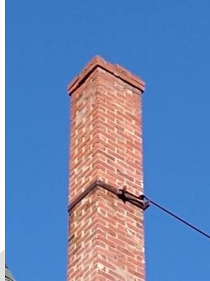
West side chimney with metal brace
