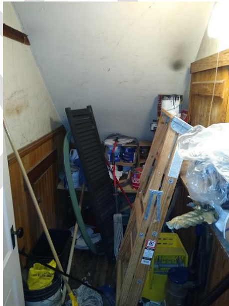
Former ticket booth under stairs to second floor
