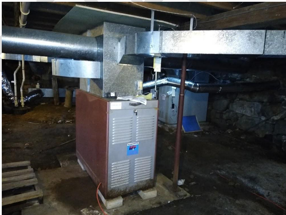
Existing hot air furnace that provides heat to the 1 st floor
