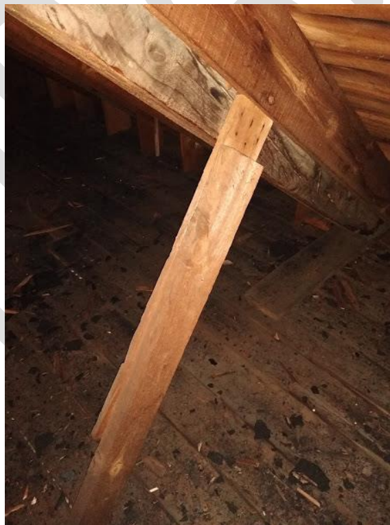
Additional wooden "make do" brace and additional rafter under original roof rafter
