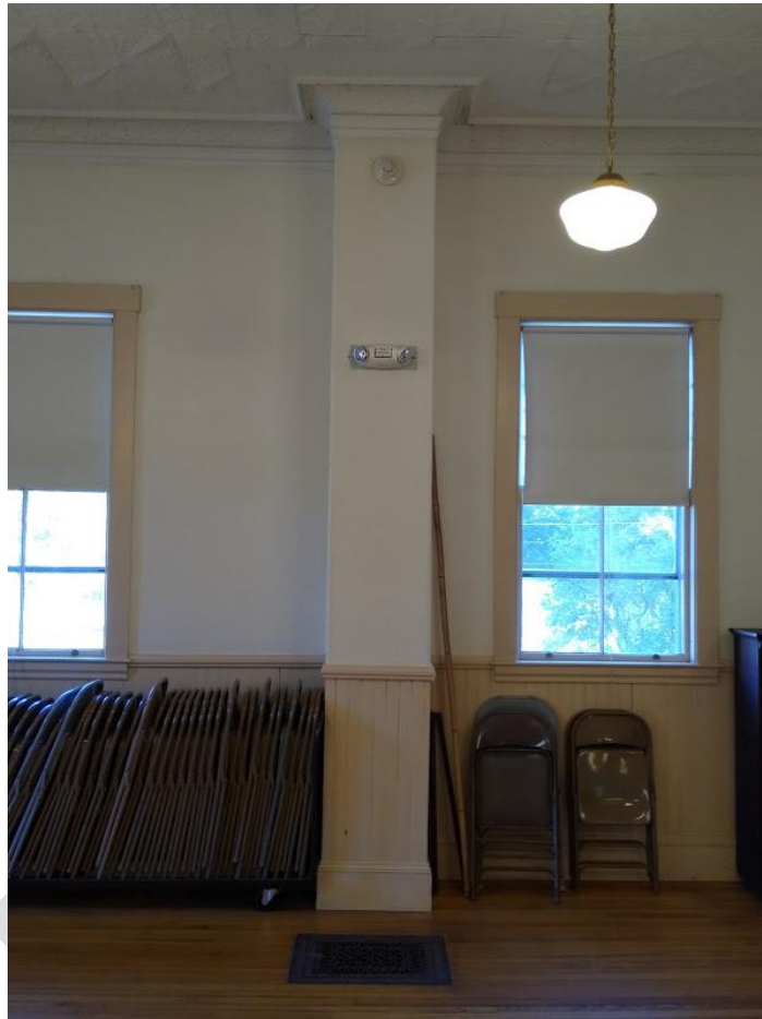
Looking east, original covered chase way for duct work to ceremonial room above. In the fore ground original, currently utilized, hot air grate
