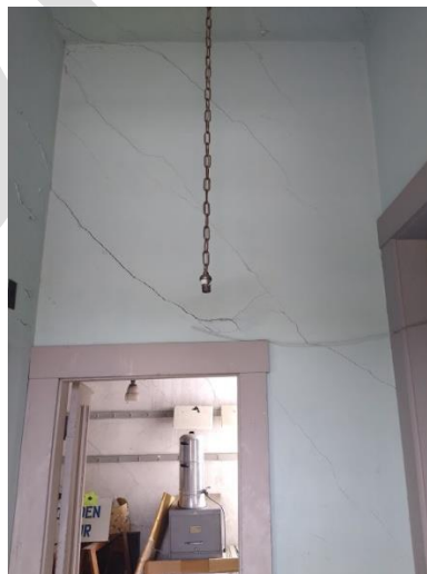
Stress cracks in plaster in landing at stairway looking south
