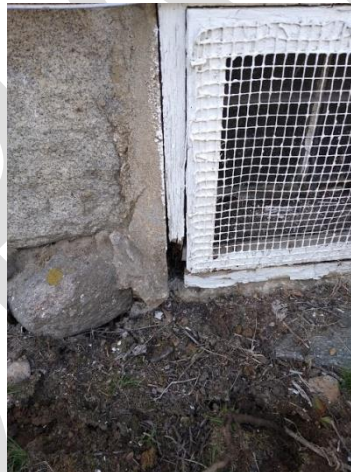
East side rotted basement sash frame
