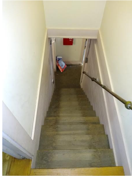
Stairs to south exit looking down from kitchen
