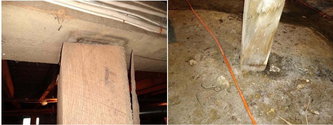
Wooden post no longer providing support for main carrier above with rotted base
