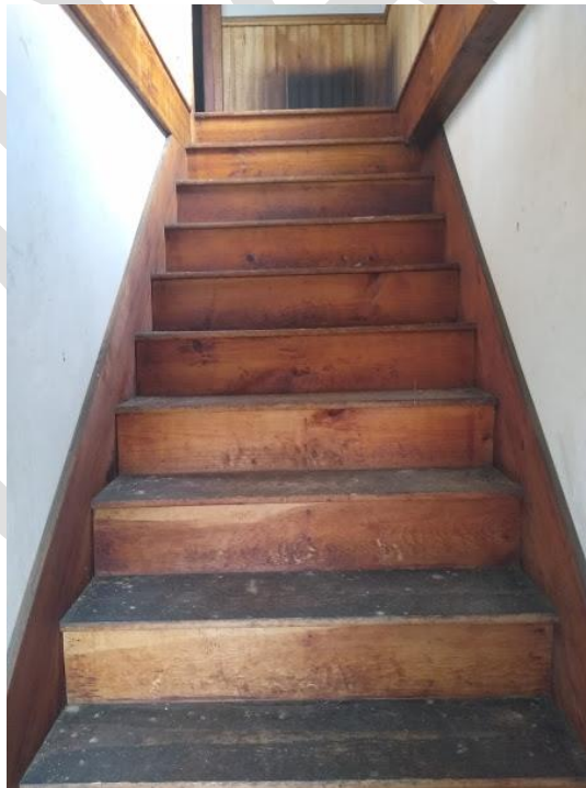
Second flight of stairs from the landing to the 3rd floor tower room
