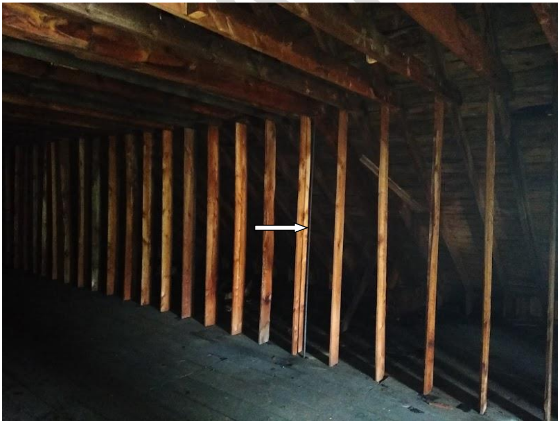
Attic framing looking southwesterly with added metal rod for partition support
