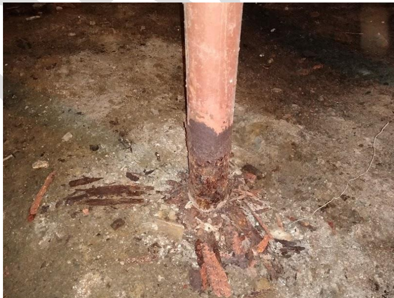
Metal column rot at base
