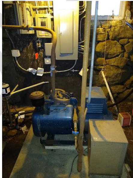
Old generator in basement
