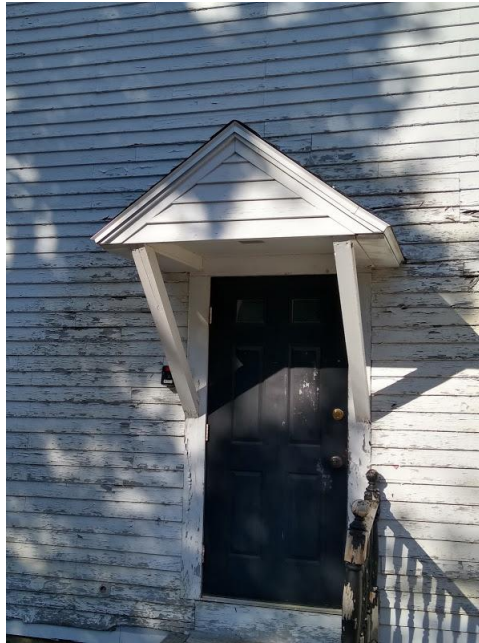
South entry roof system
