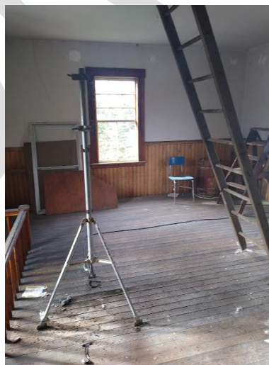
Tower room looking west with ladder to attic space above
