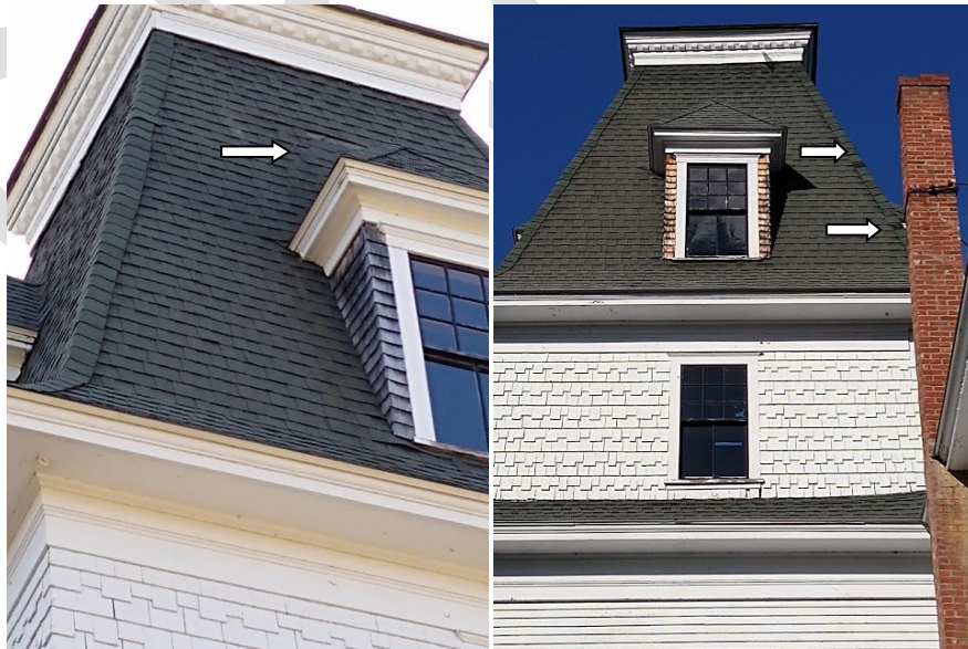
North side of tower missing shingles
