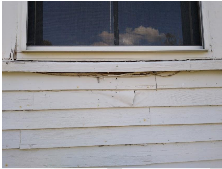
Deteriorated East side 1 st floor window sill
