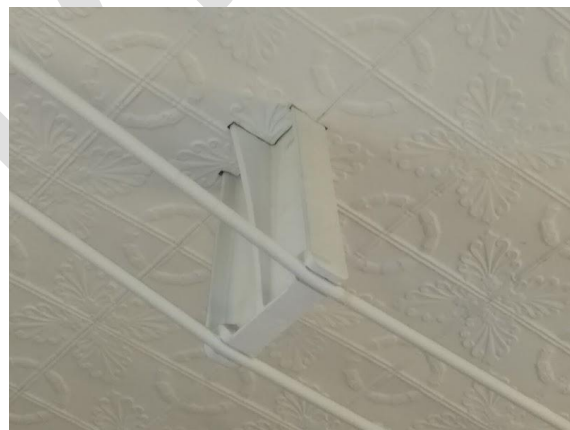
Close up of steel truss hanging down from ceiling
