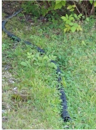
North side sump pump discharge hose
