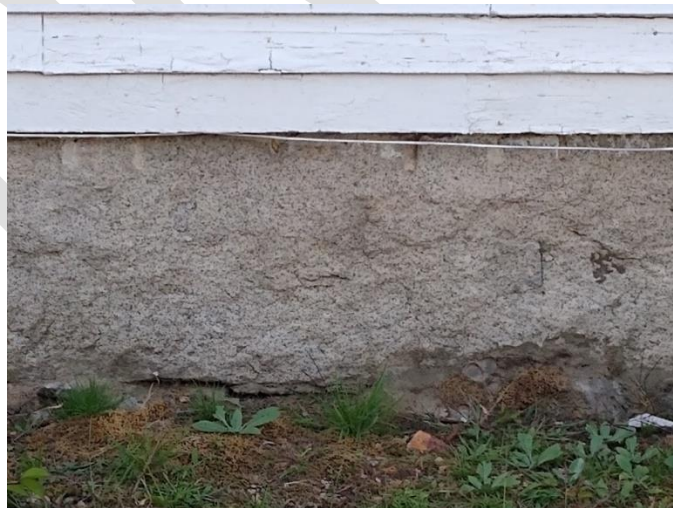
Split cut granite east side
