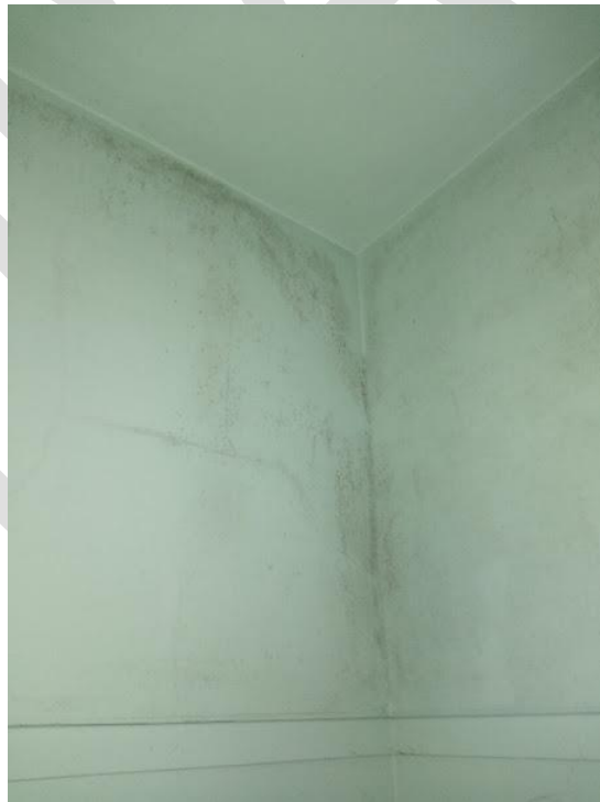
Walls and ceiling of bathroom showing surface mol
