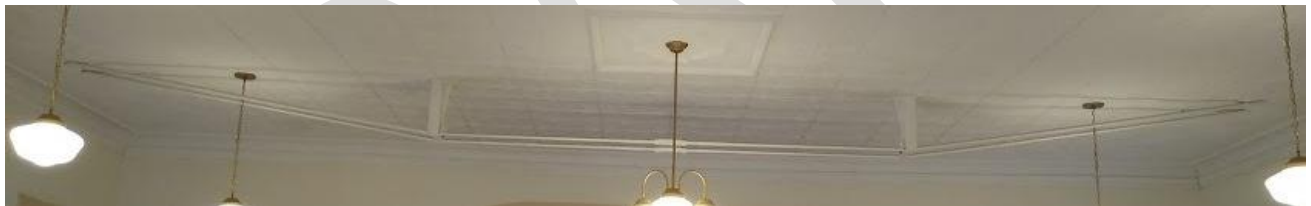
Truss system hanging down from ceiling in auditorium
